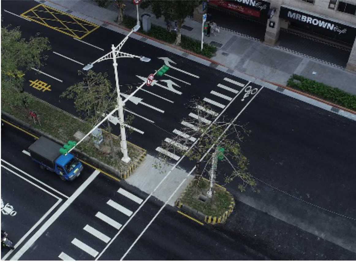
Figure 1: Multi-functional pole, pedestrian island and crosswalk
