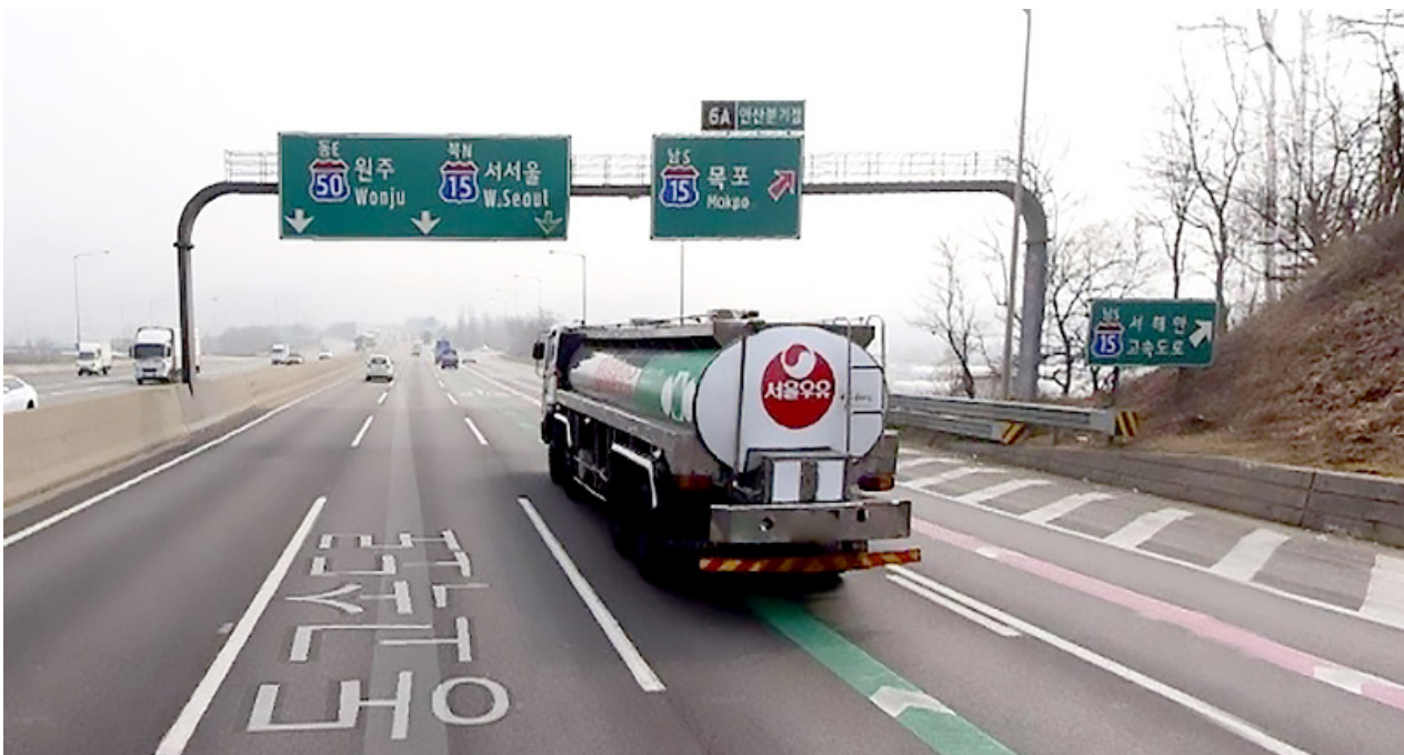
Figure 2 Ansan Junction on West Coast Expressway, the No. 1 Color Guide Line in South Korea (Naver Map Screen Capture)
