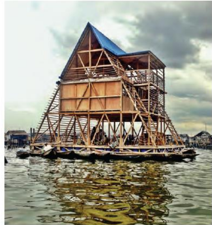
Makoko Floating School , prototype structure for the coastal water community of Makoko, Nigeria. The triangular A-frame is an ideal shape for a floating object due to its low center of gravity, which provides stability even in extreme weather conditions. Green buildings play a significant role in building resilience against future climate change and natural disasters. © NLÉ Architects
